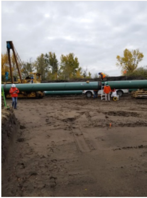
Sept 21/18 Description & Location KP- 817+789 Photo taken facing north Workers pre heating the pipe for the internal welding
