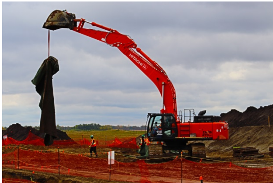
Sept 21/18 Crews were disassembling the cleaning station as it is no longer required in that area Excavator removing Caepla carpet
