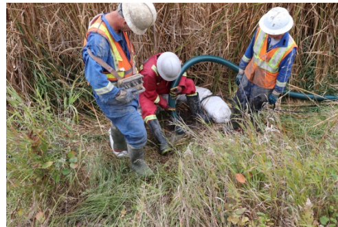
Sept 19/18 Description & Location: SSKP 899+550 Workers with SA Energy and Badger Cleaning the seeping fluid on surface Using water and suction hose to clean Picture taken in Black Creek
