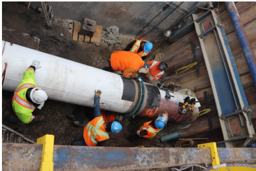
Sept 22/18 Description & Location: SSKP 825+490 Seasonal Marsh Class 3 Wetland Complex MB-1051b Tundra Bore/Trench Box/Welders Pipe clamps used to line up pipe (blue)
