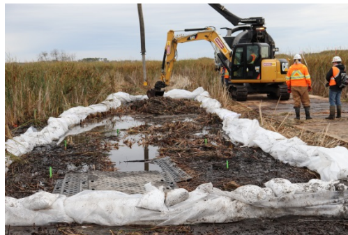
Sept 20/18 Description & Location: SSKP 840+727 Environmental Clean-up Mini Excavator digging contaminated soil Hydro-Vac in background facing west Sandbags used to contain spill
