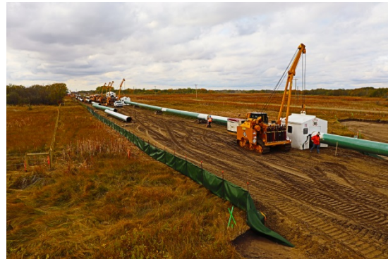
Sept 21/18 Pipe Gang and Poor Boy Welding crews working in a Semi-Permanent Marsh Class 4 Wetland Complex MB-1039 Phot facing NW
