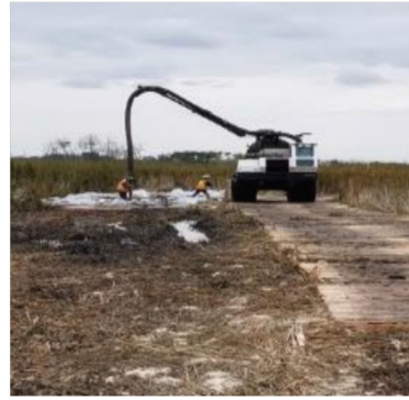
Description & Location KP-841+100- Facing E Worker's cleaning swamp with hydro-vac
