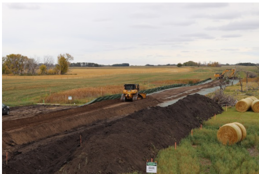
Sept 19/18 Description & Location: SSKP 850+100 Seasonal Marsh Class 3 Wetland MB-073 Dozer and Excavator building ramp through wetland complex photo facing NE
