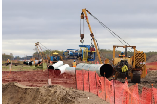
Description & Location: SSKP 818+050 End Prep crew beveling pipe ends Facing east
