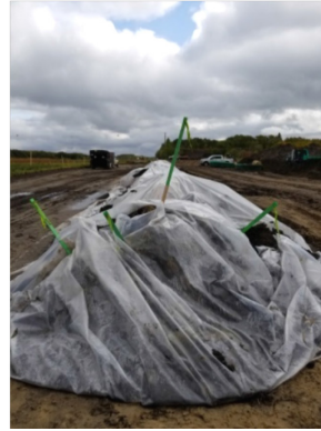
Sept 21/18 Description & Location KP-841 + 553 Soil wrapped and covered with poly from the wetlands west of SF # 28. Photo facing west
