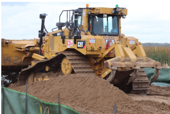
Sept 21/18 Semi-Permanent Marsh Class 4 Wetland D6 Dozer pushing sand on wetland ramp Close to environmental spill site Photo facing NW
