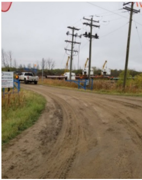
Sept 22/18 Description & Location KP-819+400 148 west Side booms moving the welders shacks to SF # 13 east. Photo taken facing south
