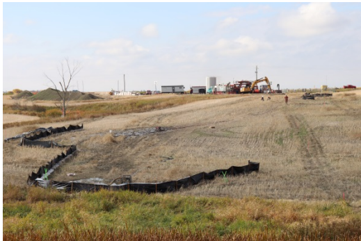
Description & Location: SSKP 899+450-Facing west Black Creek boring crew Some fluid released through cracks Clean up crew doing good job containing it
