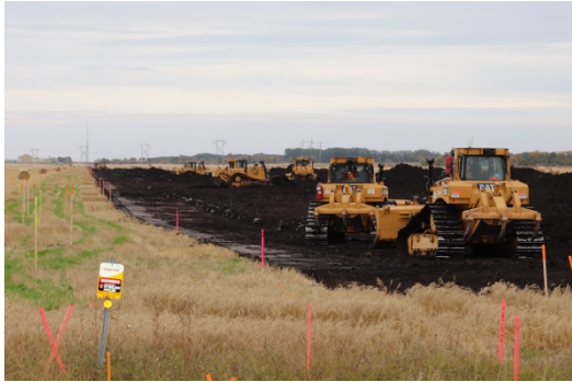
Sept 19/18 Description & Location: SSKP 870+550 Grade crew stripping and piling soil Dozers pushing soil and Power dozer Pink stakes beside dozers are 5 m buffer Photo facing east
