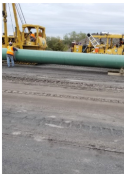
Sept 20/18 Description & Location KP-815-100 bone yard Side boom moving the pipe for the welders to start welding Photo taken facing south.
