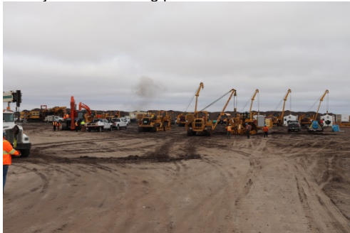
Description & Location: Bone Yard-Facing North Very congested area Unloading side booms and automatic welders Pipe Gang getting prepared
