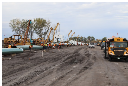
Sept 19/18 Description & Location: SSKP 812+700 Main gang welding mainline facing west Very congested biggest crew on job Preheaters, Automated Welders Root pass, Hot pass, Cap and Rotoscan
